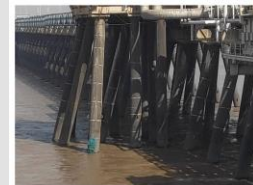
Jetty Pile Casing or Pipe Rack Inspection
