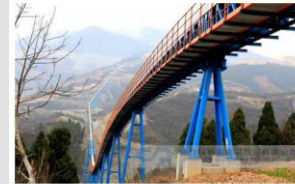
Conveyor Super Structure Inspection
