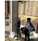
UPV Testing on column
