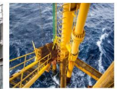
Offshore Riser Pipe Inspection
