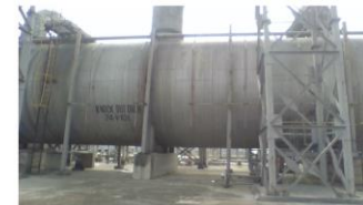
Horizontal Vessel External Shell Inspection
