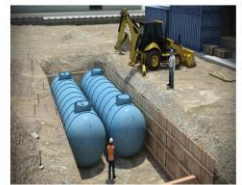
UG Tank Internal Inspection
