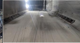
Boiler Tube Inspection
