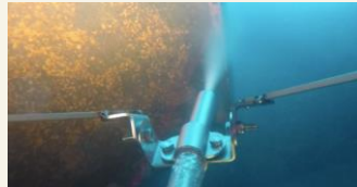
Spot Cleaning of Marine Growth
