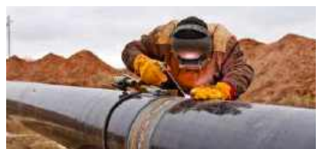
Construction, Utilities & Pipeline Laying
