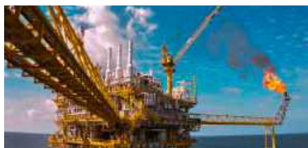
Offshore Industries like Subsea platforms, Jetty Piles etc.
