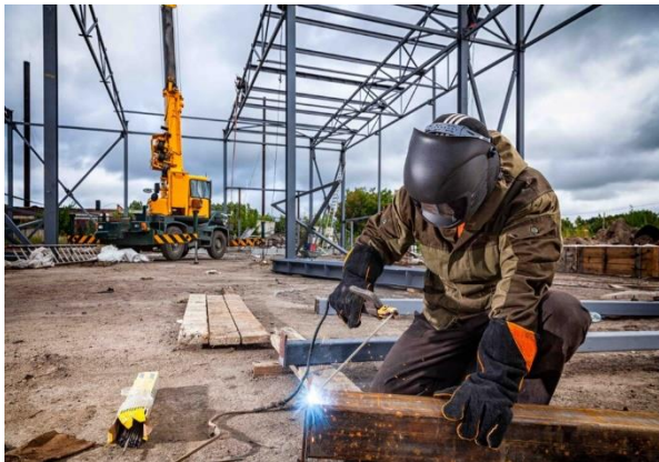
Welding Inspection & Certification
