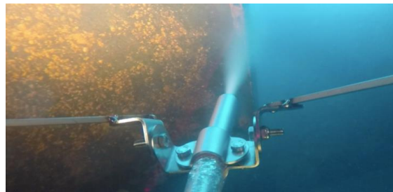
Spot Cleaning of Marine Growth
