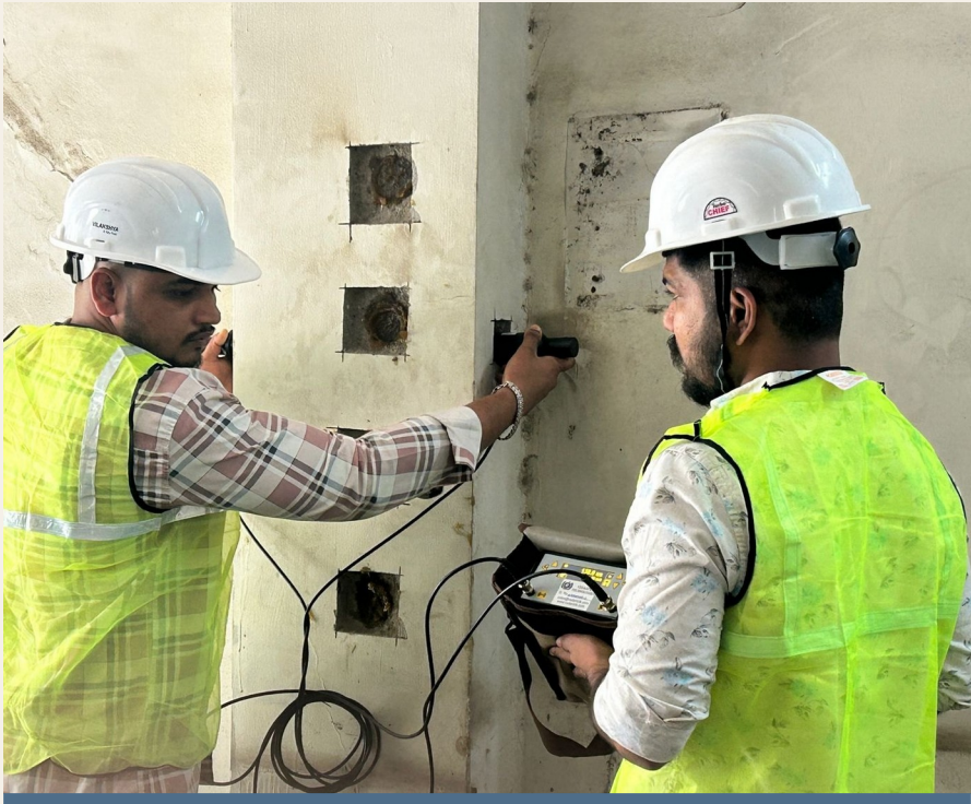
UPV survey on a concrete column, TCR field team
