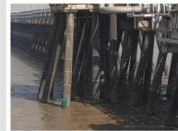
Jetty Pile Casing or Pipe Rack Inspection
