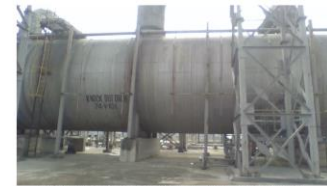
Horizontal Vessel External Shell Inspection
