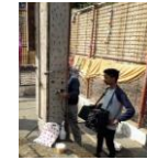
UPV Testing on column
