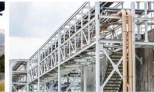
High Rise Pipe Rack Inspection
