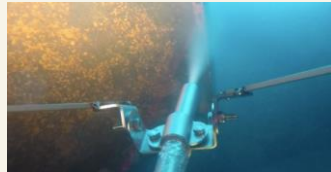
Spot Cleaning of Marine Growth
