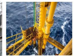
Offshore Riser Pipe Inspection
